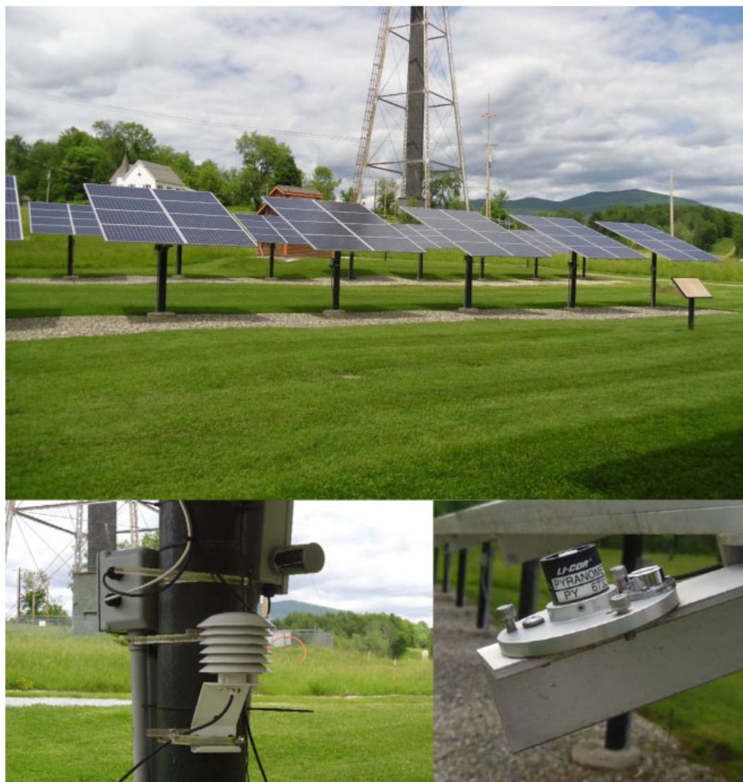
Figure 1. Green Mountain Power Solar array (top), air temperature sensor (bottom left), and (bottom right) pyranometer measuring the solar flux orthogonal to the panel.
