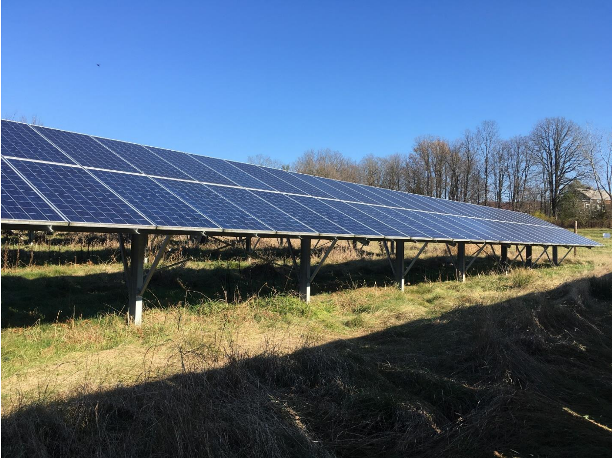
West Haven Solar Array
